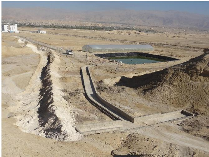
Photo 1 Rainwater harvesting system developed in an arid environment
