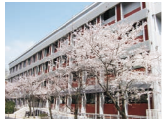
Research Building Reinforced concrete, one floor underground and four floors above ground built between 1964 and 1967. Aseismic repair in 2009 Northern Campus of Kyoto University, Kitashirakawa Oiwake-cho, Sakyo-ku, Kyoto
